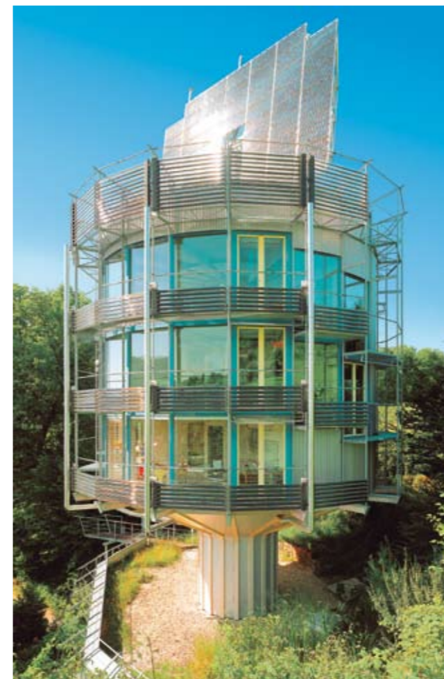
Das Heliotrop® in Freiburg
