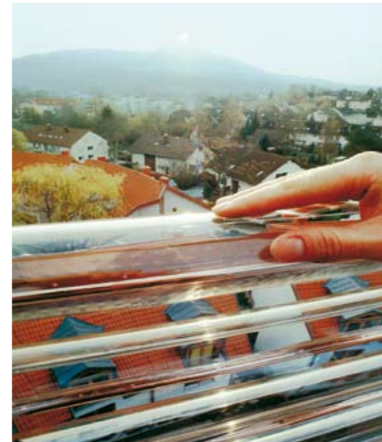
Solar-thermal collectors as balustrade
